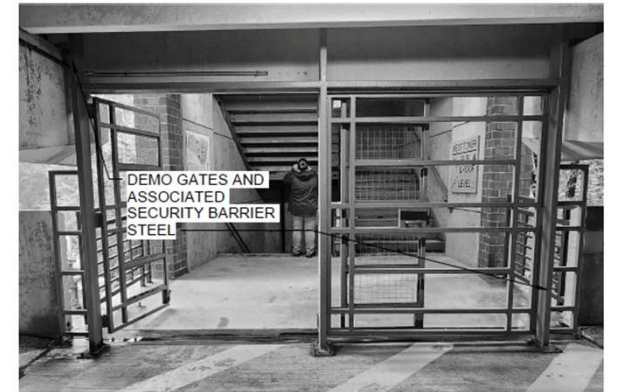
2 PHOTO - WEST STAIR, LEVEL 4 (LEVELS 2 & 3 SIMILAR) A-403 SCALE: NONE
