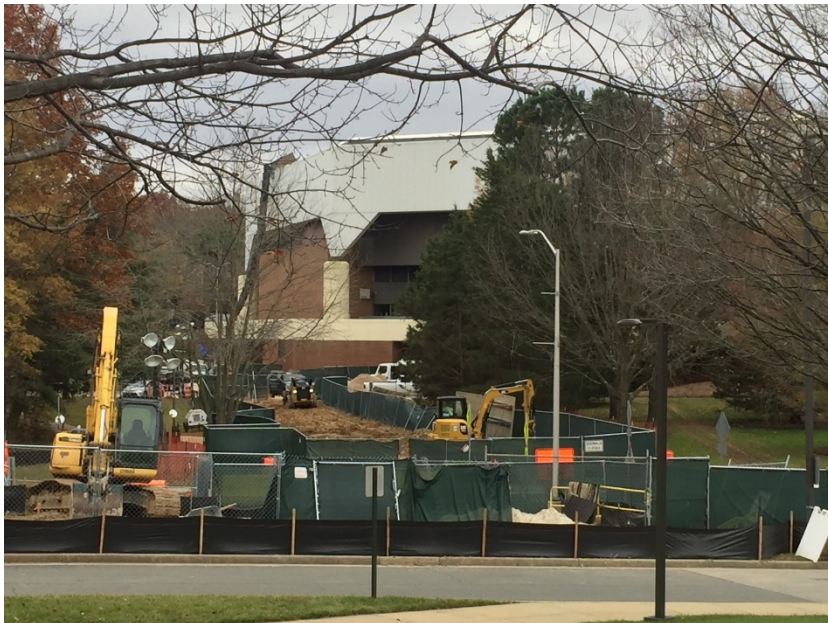
Phase 1C – Existing Chilled Water S/R replaced to EBA
