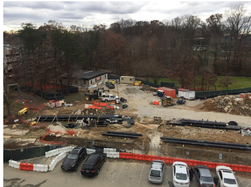
Construction Laydown area in site of removed Student Apts.
