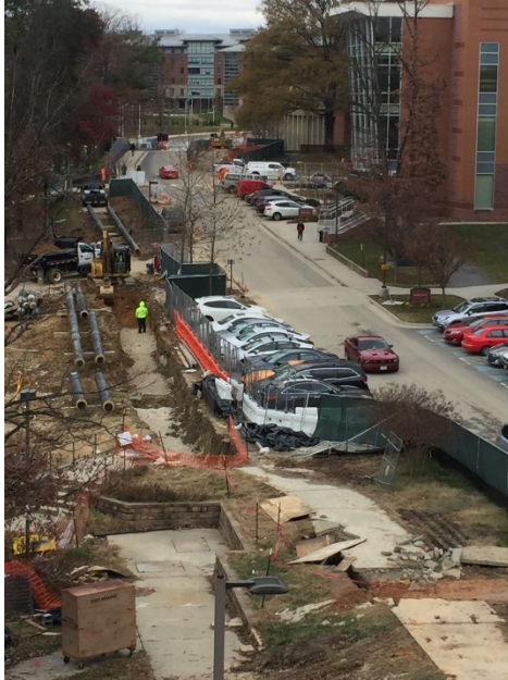
Phase 1A – New Chilled Water loop at Aquia Lane
