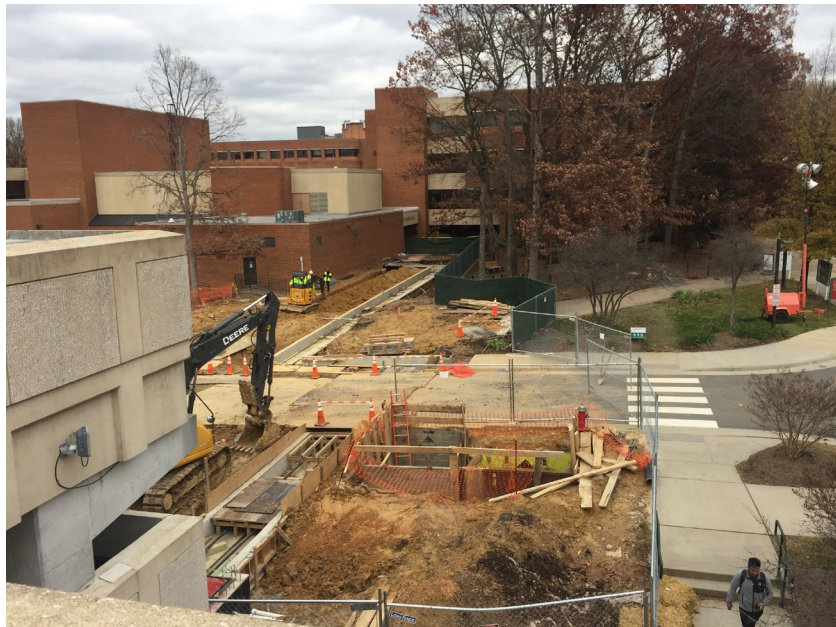
New Chilled Water, High Temp Hot Water and Domestic
