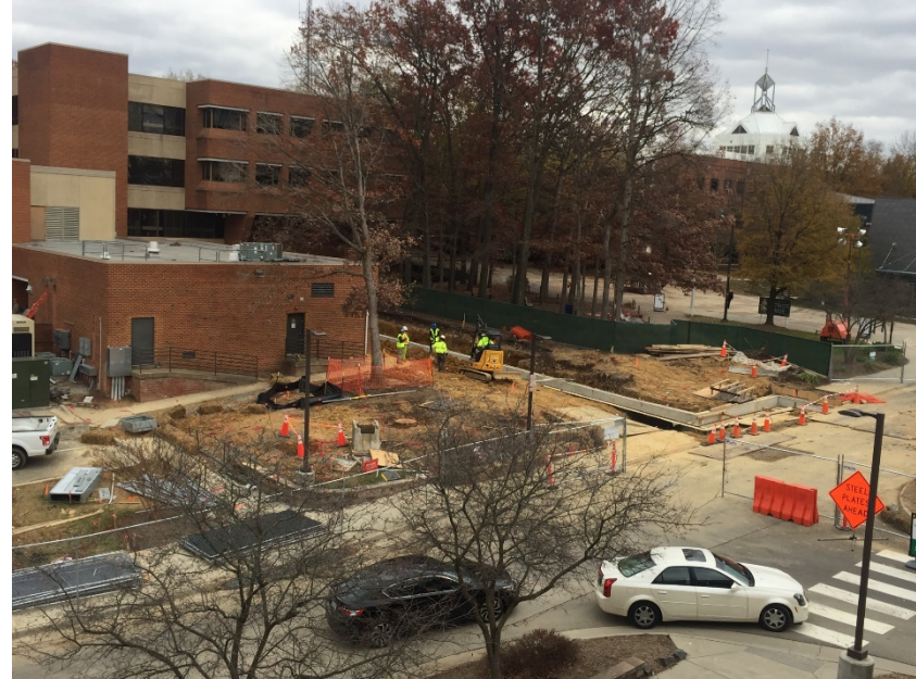
New Transformer and Generator for Harris Theater
