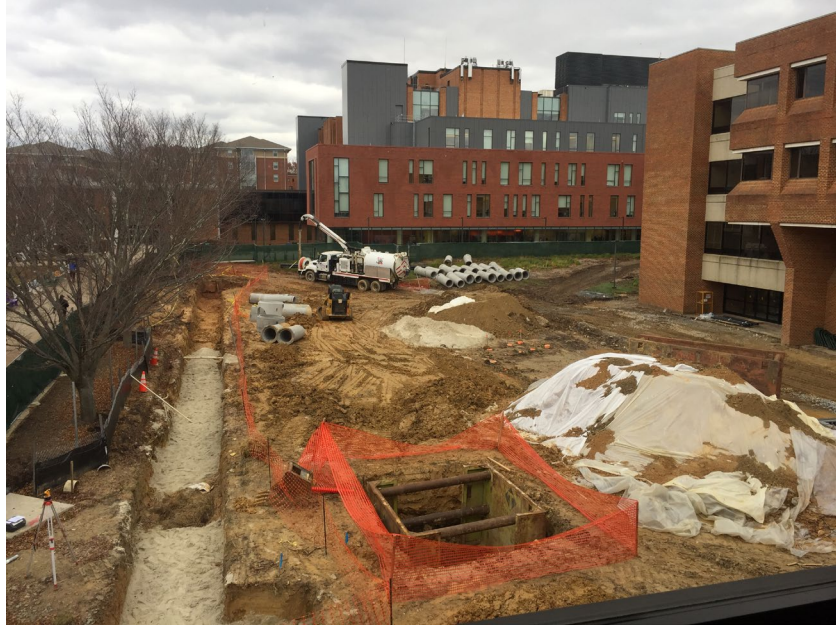
Relocation of site utilities at new building footprint
